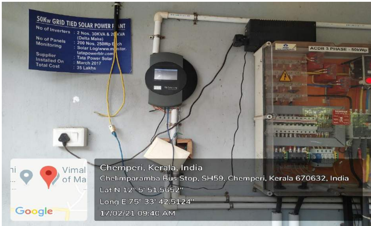
Figure 7 & 8 showing solar power supply
